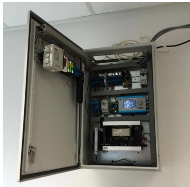
Figure 3 – Control cabinet of BINGO! with power supplies (black box, bottom), exposure controller (black unit door), DCF clock (grey box middle row left), chopper wavegenerator (blue box), GSM I/O module (grey box door).
