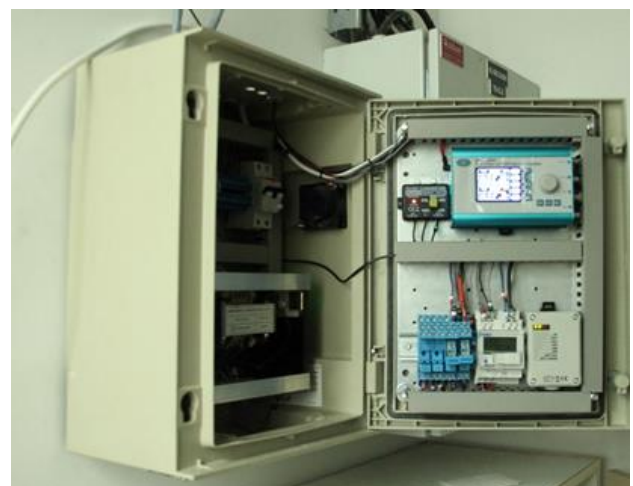
Figure 4 – Control cabinet POGLED. Power supply (black box, bottom), exposure controller (grey box, door, lower row, center), chopper controller (blue box, door), GSM I/O module (door, bottom, right).
