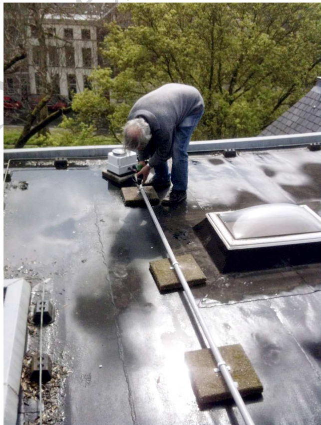
Figure 4 – Installation on the roof of the Old University Observatory.
